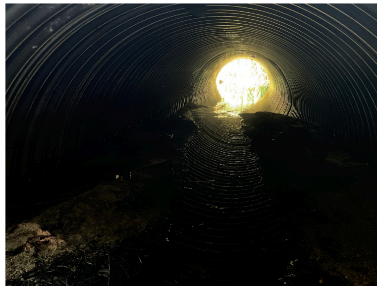
Looking Downstream Through CMP
